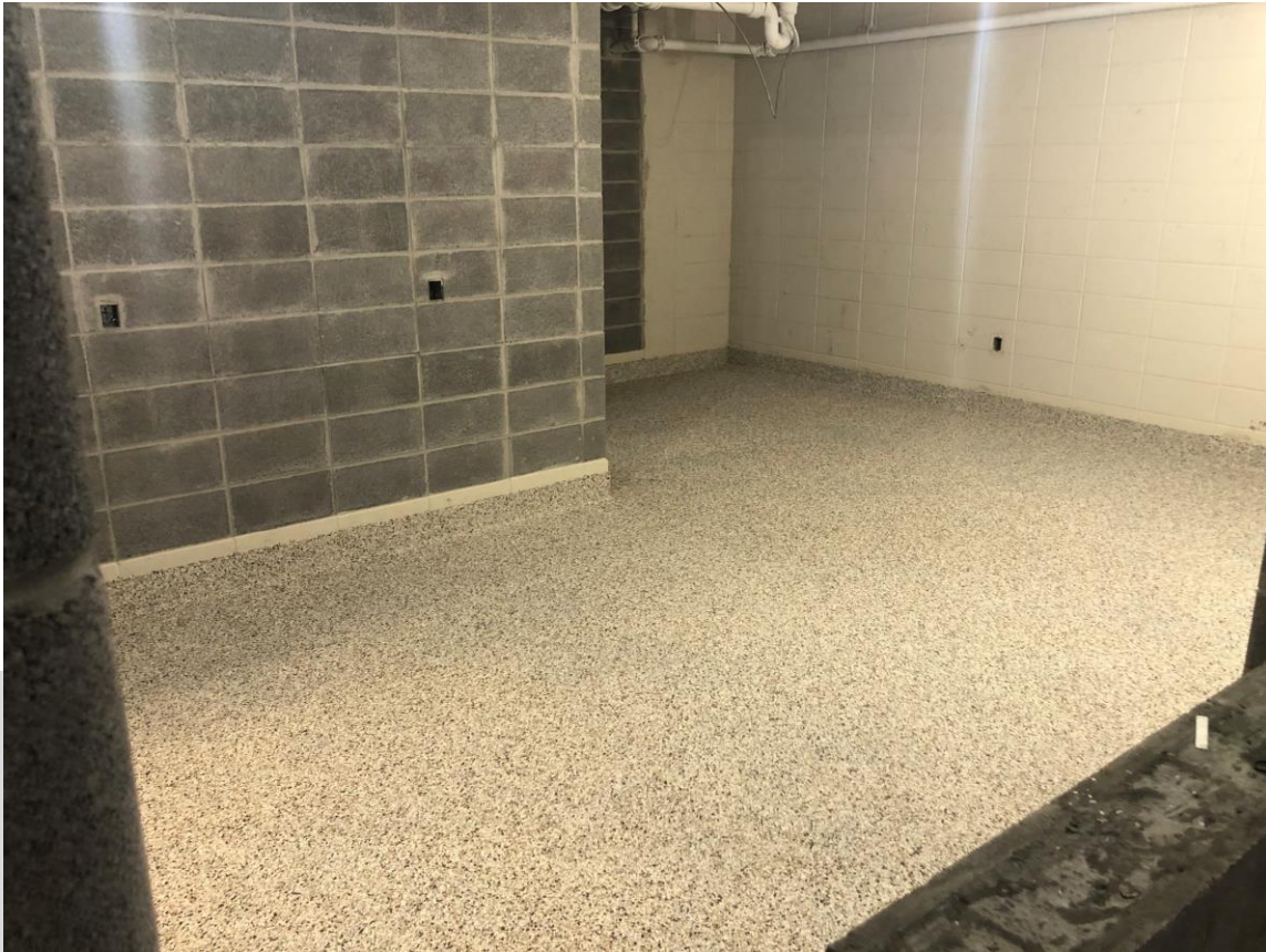
Epoxy Installed in Concession Stand at Performance Gym
