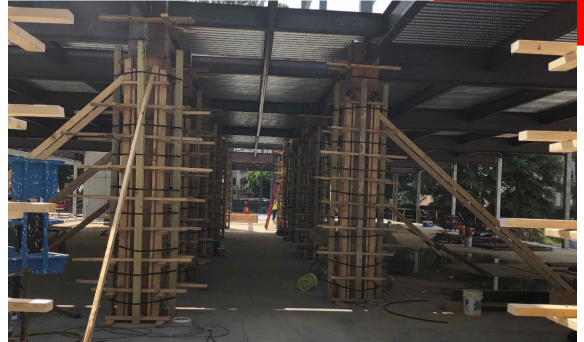
Second floor interior columns formed
