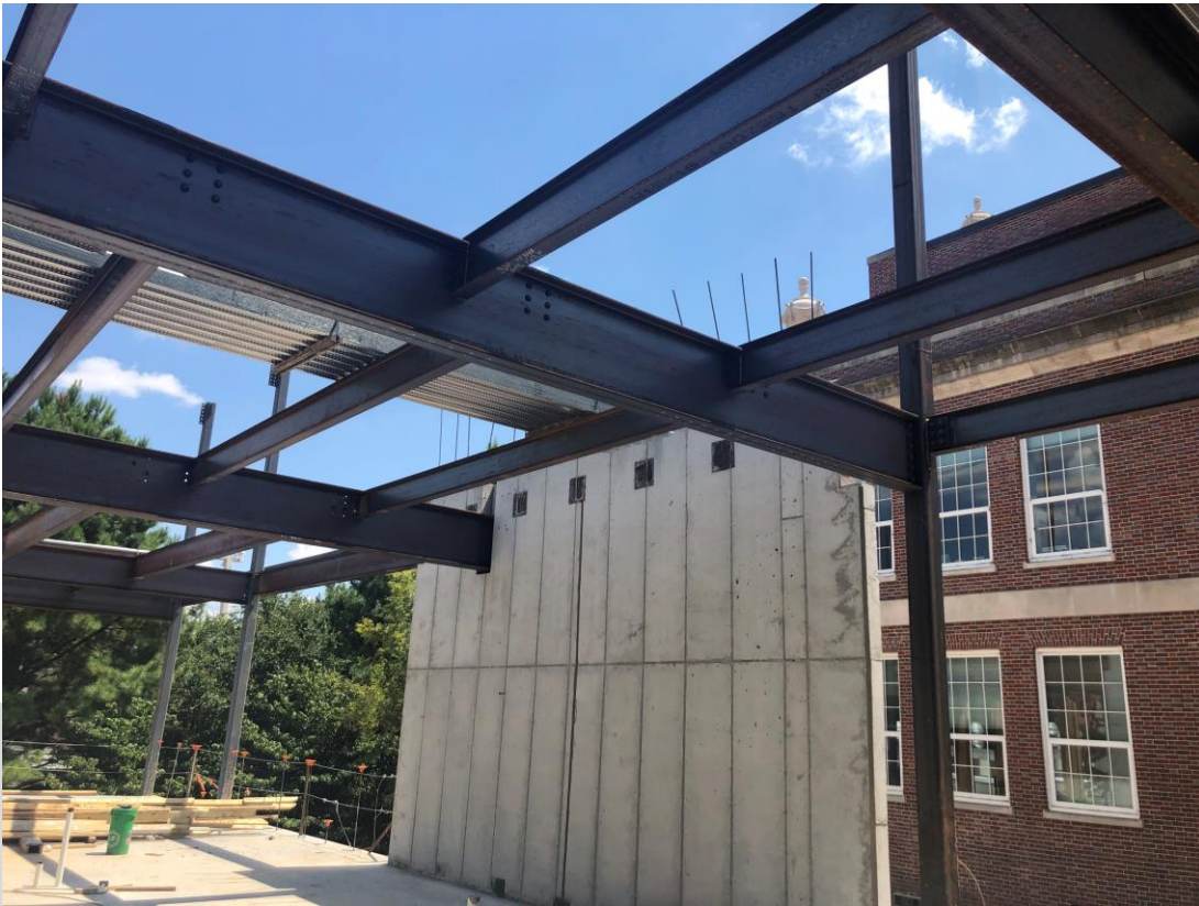
Beams tied into Second Floor Shear walls
