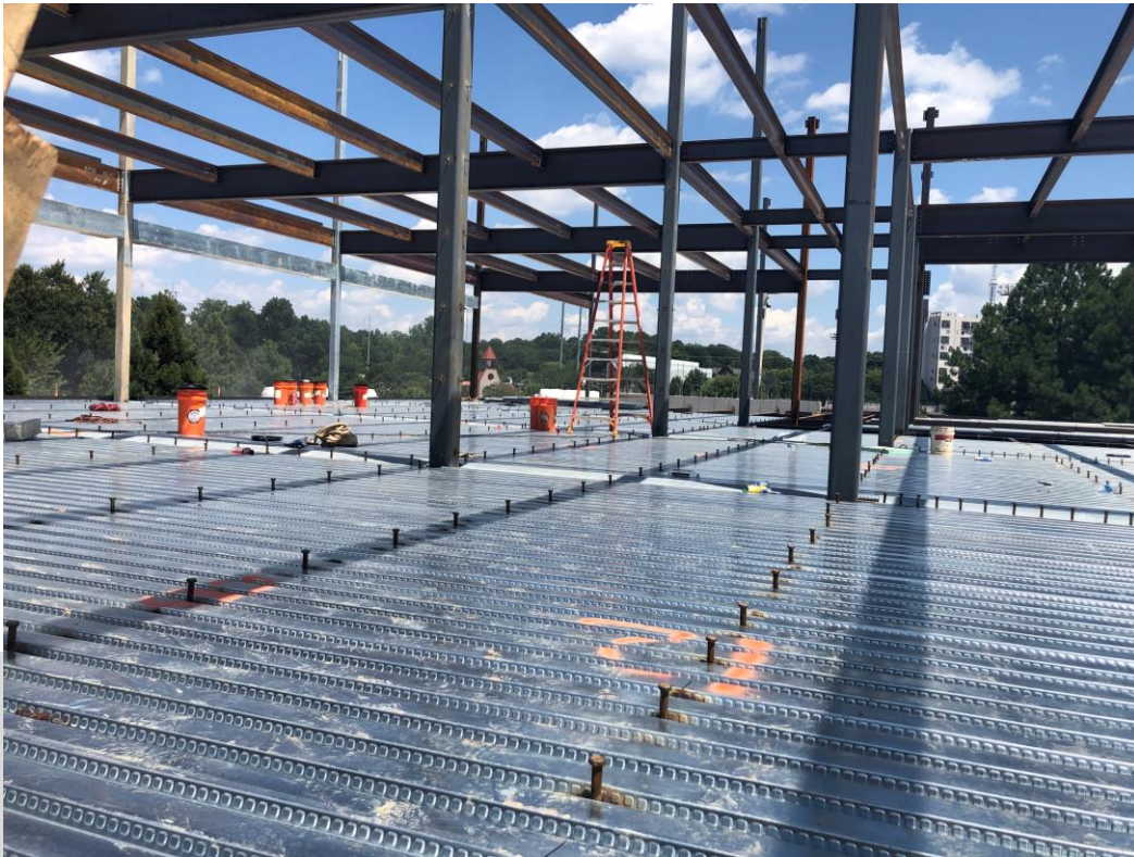
Third Floor Decking Installed
