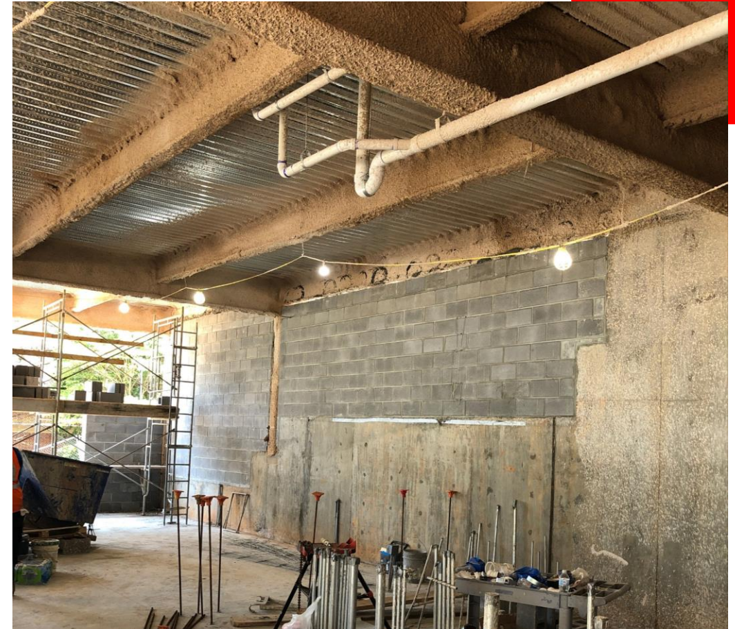
CMU Installed at SE Wall
