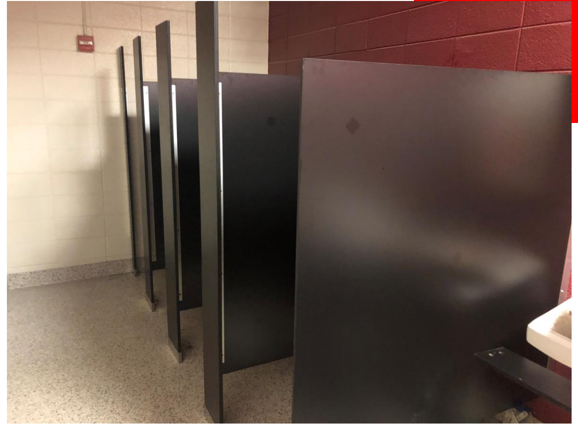
Toilet Partitions installed in Performance Gym Bathrooms
